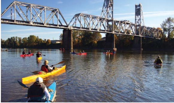
Kayakers under Union Street Railroad Bridge
